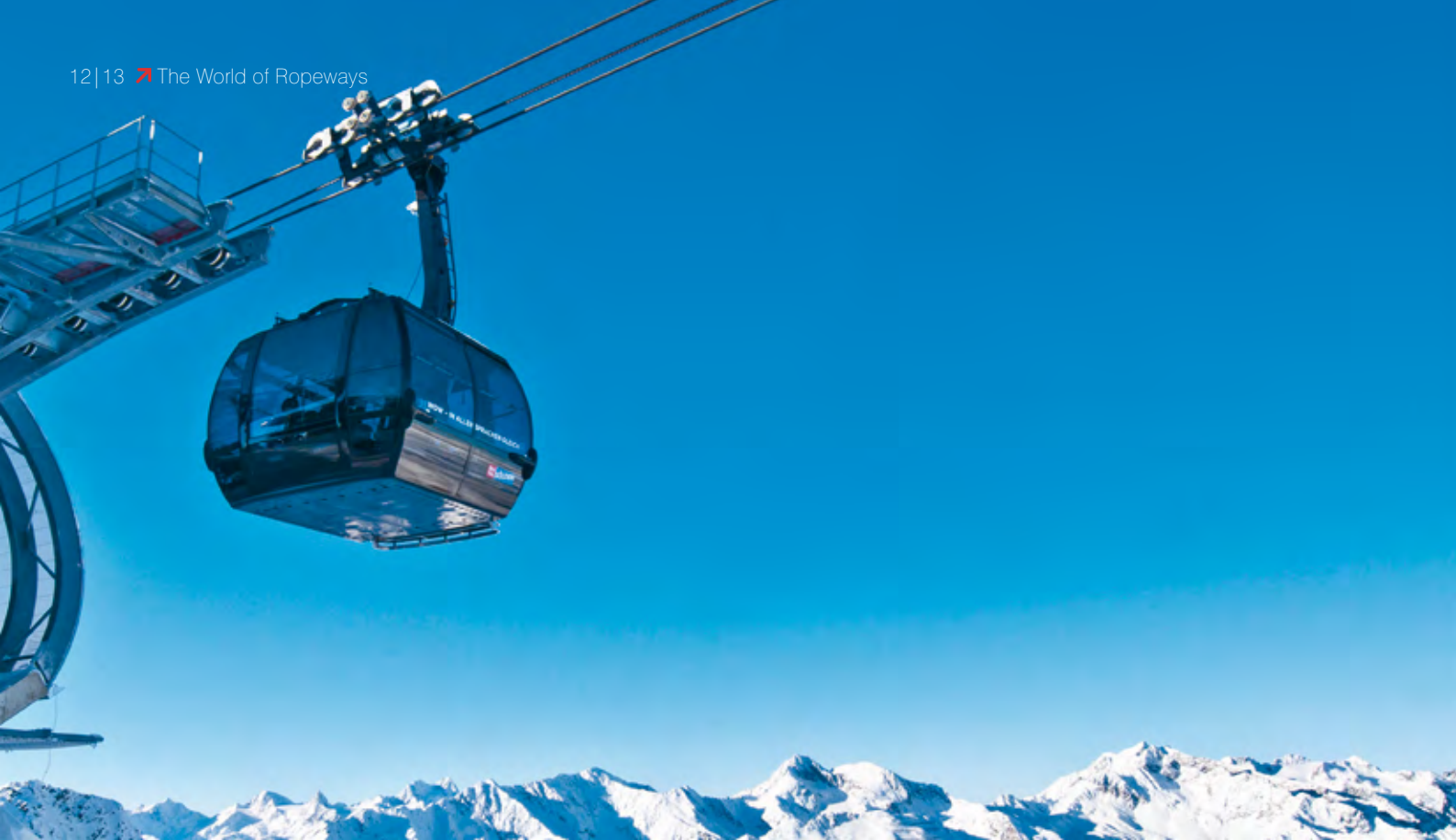
3S gondola lift – Sölden, AUT
